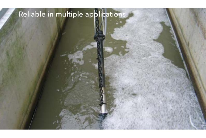
Conductivity is a well recognized and often indispensable parameter of stateof-the-art water, wastewater and industrial process analysis. Continuous measuring systems are employed to monitor the salt load of the influent in wastewater treatment plants, to control quality of drinking water and ultra-pure water or to determine non-specific contaminants in industrial processes.
