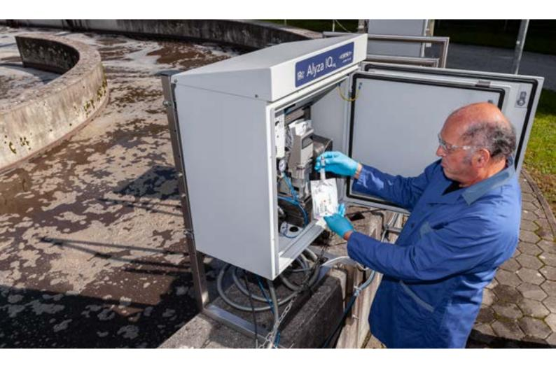
In the wastewater treatment industry, there has been an increased need for on-line measuring analyzers justifying their market presence next to less expensive in-situ sensor systems. Especially when it comes to high-precision water analyses, for example in the monitoring of the discharge in sewage treatment plants requiring automatic calibrations and/or adjustments as well as standard DIN methods for analysis, analyzers are necessary.
