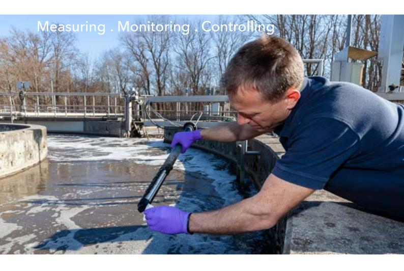
Reliable and continuous measurements of dissolved oxygen have become vitally important in many areas of the water/ wastewater treatment facilities. The availability of accurate and real-time measured concentrations is an absolute requirement for process monitoring and dynamic process control to ensure an efficient plant operation.
